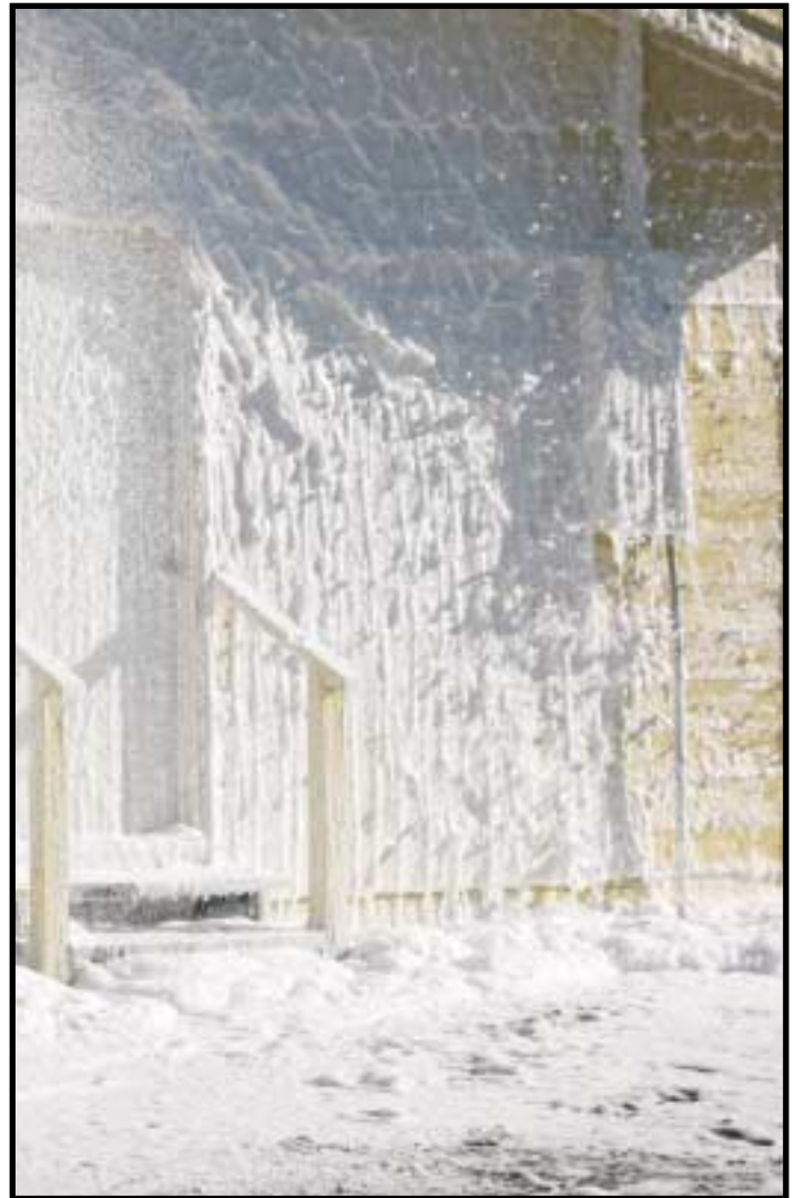
Foam blanket being applied to a house
